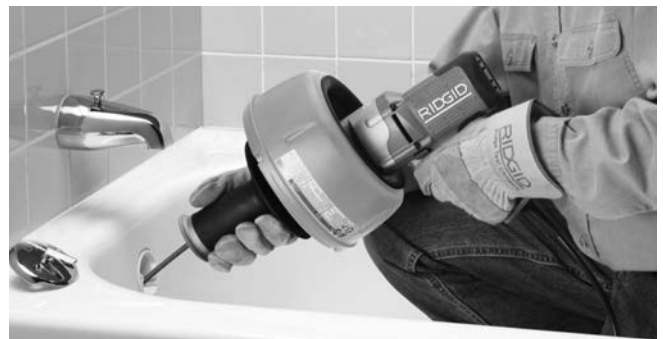
Figure 9 – Push Cable Down Drain Line
