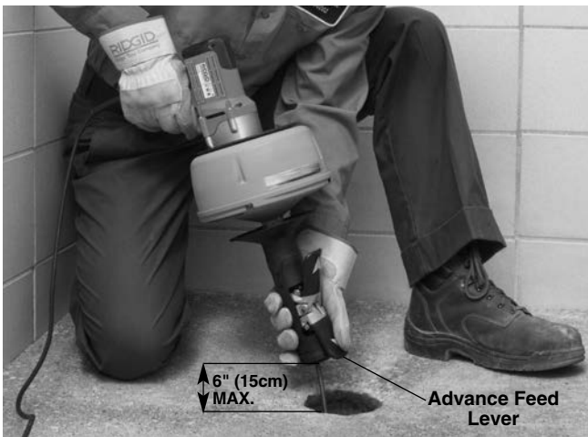
Figure 10 – Feeding Cable With AUTOFEED
